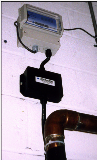
TWT-5C8-402/2" controller with TWT-CSE-0227 copper pipe signal enhancer. Onsite solenoid application, on 2" copper pipe.
